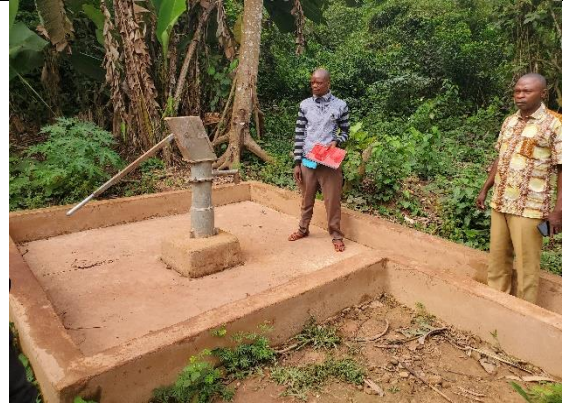
Forage CFCL Barumbi Tshopo
