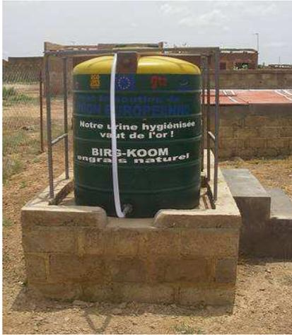
Figure 12. Above-ground plastic urine storage tank in Ouagadougou, Burkina Faso as part of EU-funded CREPA project ECOSAN\_UE (source: S. Rüd, 2008).
