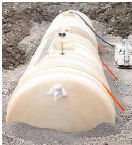
Figure 10. Below-ground plastic urine storage tanks at Kullön, Sweden during the construction process. The tanks will be covered with soil. Photo: Mats Johansson (source: Kvarnström *et al.* (2006), page 36).
