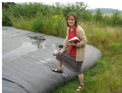
Figure 11. Urine storage tank made of a plastic bladder (3 x 150 m<sup>3</sup>) at Lake Bornsjön near Stockholm (Sweden). Photo commissioned by: E. v. Münch (2007).
