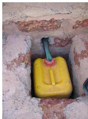
Figure 9. Low-cost solution: 20 L plastic jerrican for urine storage at individual toilet level in Ouagadougou, Burkina Faso (source: E. v. Münch, 2006).
