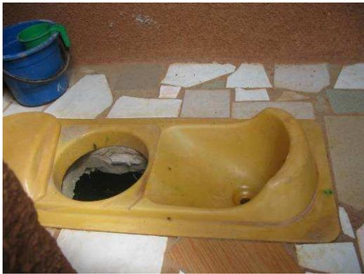
Figure 6. UDD toilet (squatting type) in Ouagadougou, Burkina Faso, installed by NGO CREPA. Source: E. v. Münch, 2006.
